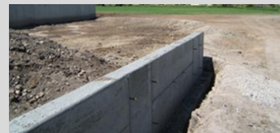
Completed Manure Bunker near Spring Creek
