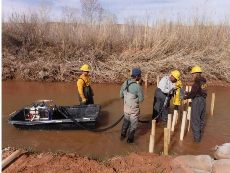
Picture of Canyon Country Youth Corps personnel installing BDA structure.
