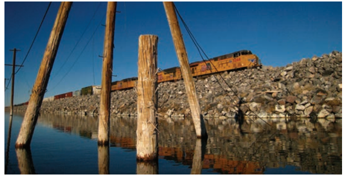
The Council has been working with Union Pacific Railroad to ensure a new causeway bridge optimizes lake flows between the north and south arm. ©Don Leonard
