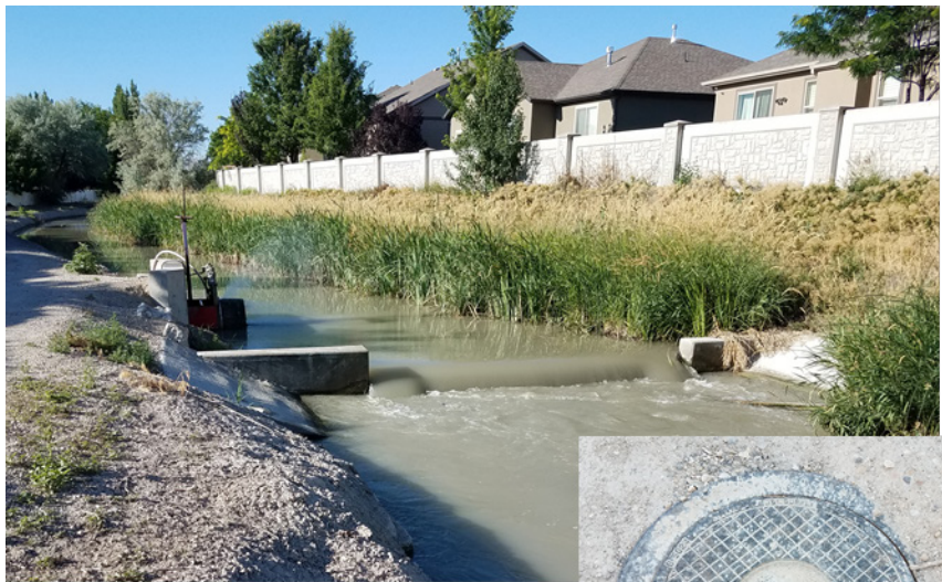
Figure 3-2. A Typical Urban Secondary Water Diversion with a Flow Meter Only at the Diversion, Salt Lake County, Utah
