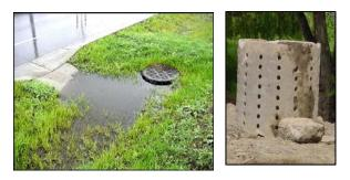
Typical UIC stormwater wells (drywells)
