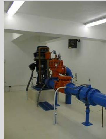
Floor Drain in Typical Well House
