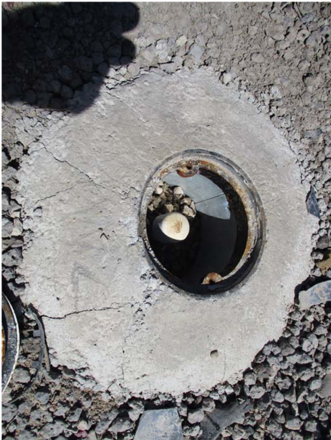
Damaged well vaults; Bottom, MW2; Top: MW3
