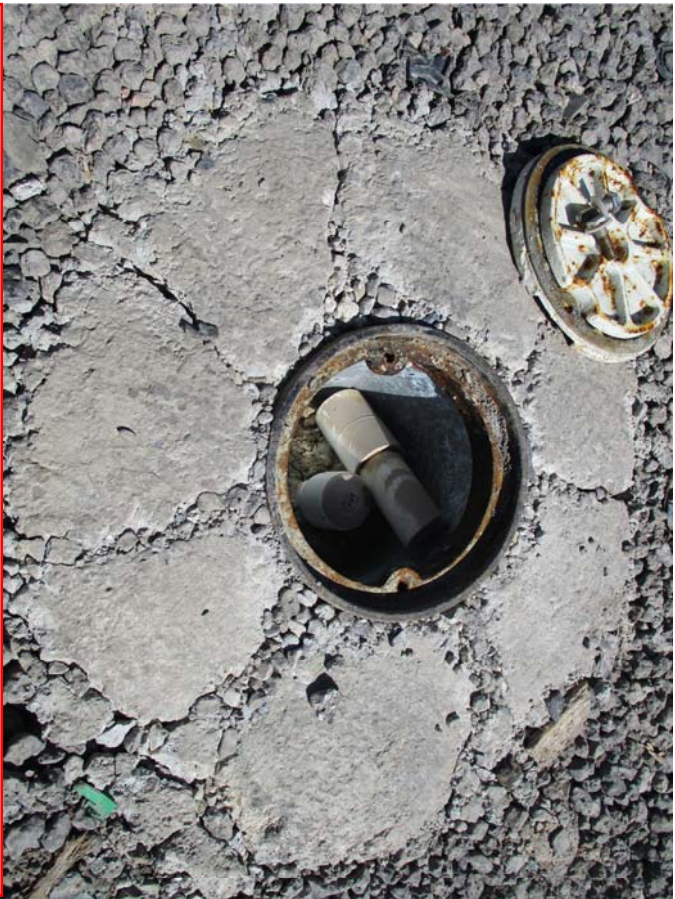
Damaged well vaults; Bottom, MW2; Top: MW3
