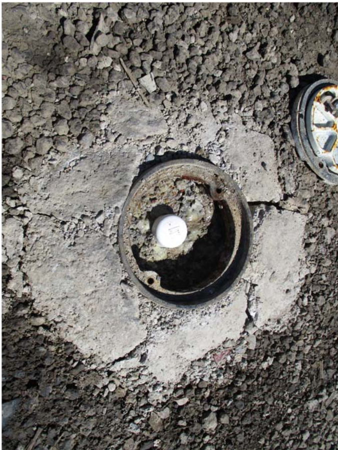
Bottom, Damaged well vault MW4; Top, Resurvey of all wells
