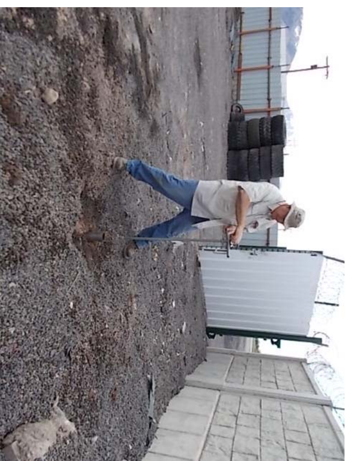
Bottom: hand augering HB8/MW1; Top: Completed MW1
