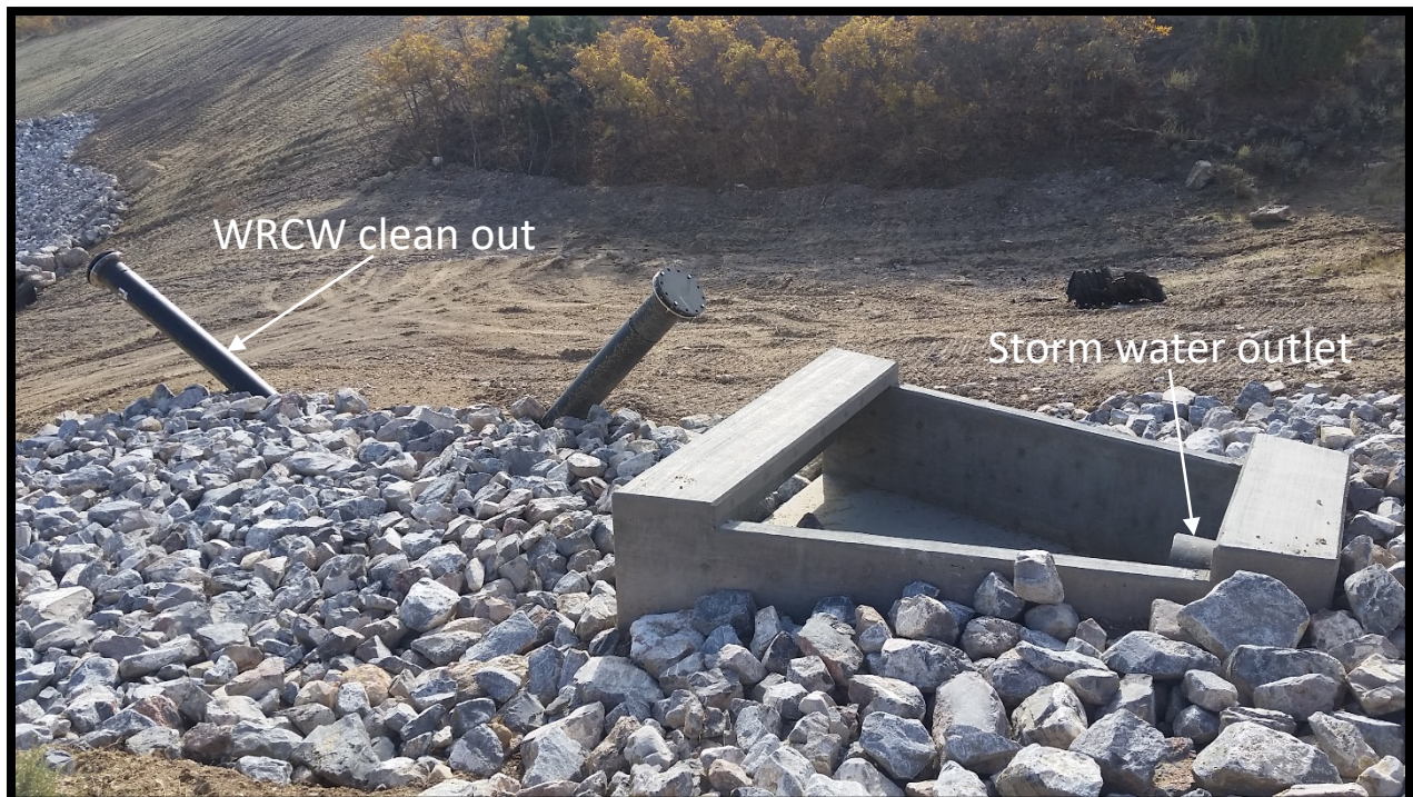
Figure 2-18. Lost Creek drainage directional boring outlet.
