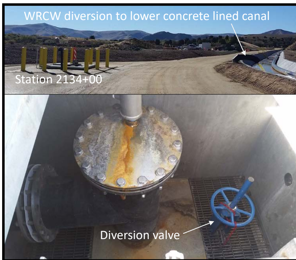
Figure 2-25. WCRW branch vault (Station 2134+00) can divert water into the lower concrete lined canal when maintenance is required at the Settling Basin.
