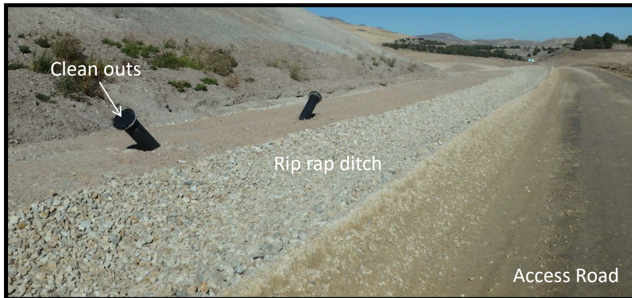
Figure 2-5. Typical toe drain showing clean-outs, rip-rap surface water ditch and the access road.
