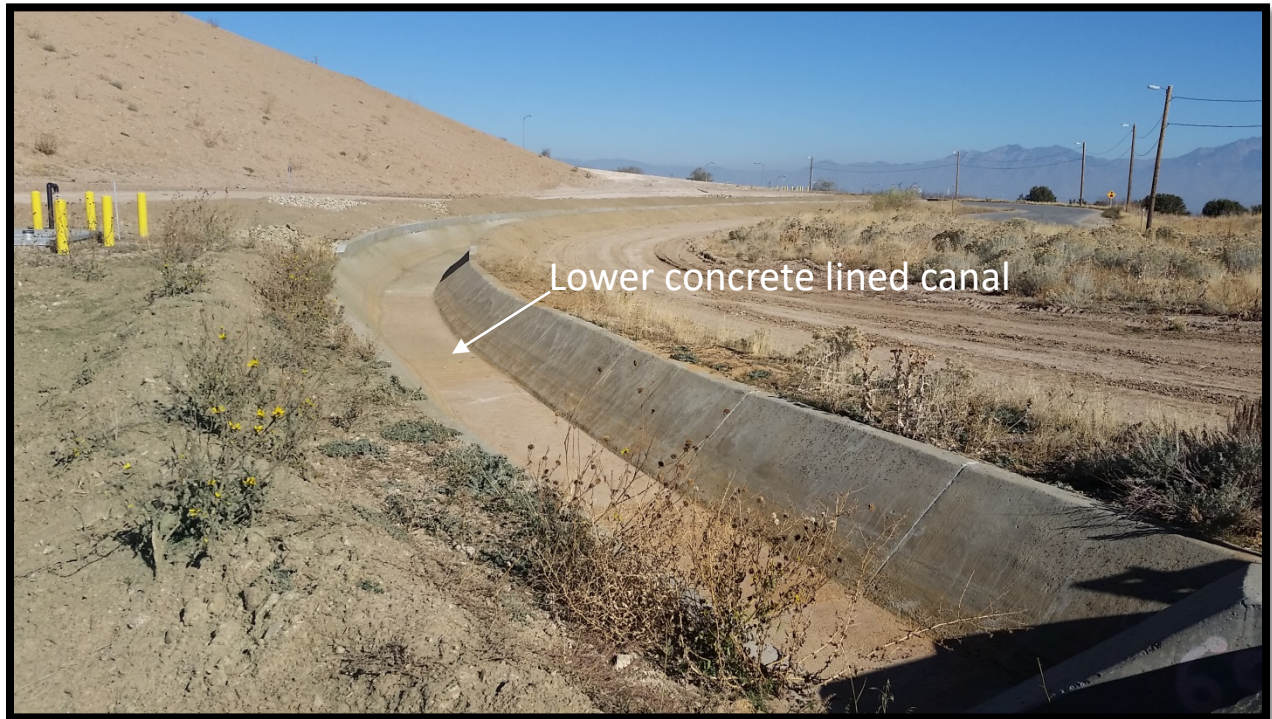
Figure 3-12. Section of the lower concrete lined canal.
