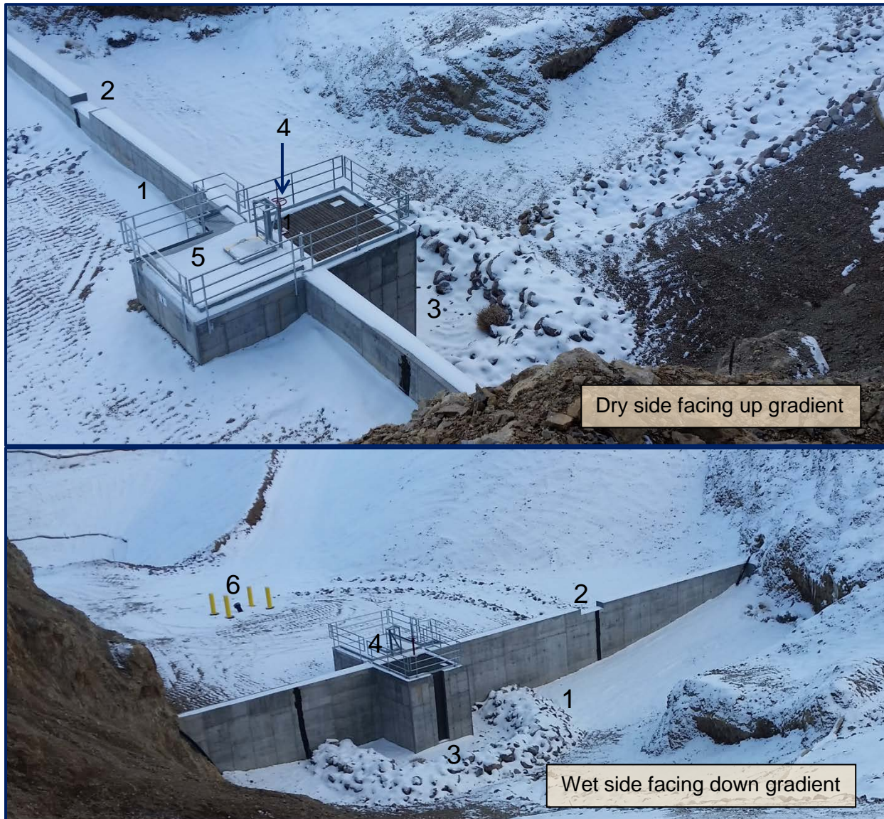
Exhibit 3. Cut-off Wall Components Illustration
