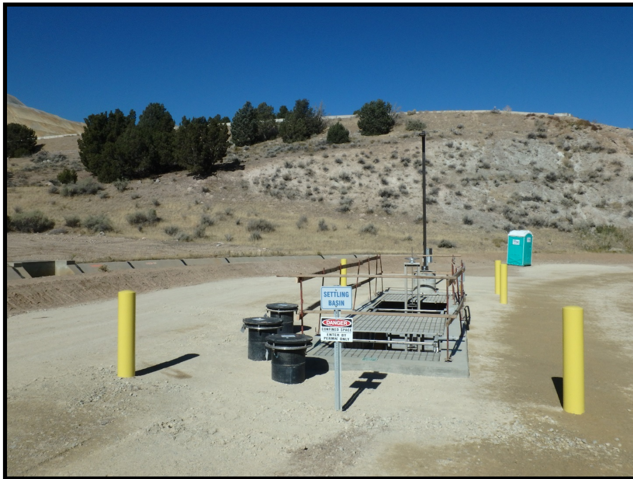
Figure 2-14. The WRCW Mainline terminates in the settling basin; from the settling basin, WRCW is conveyed to the Midas Pump Station.
