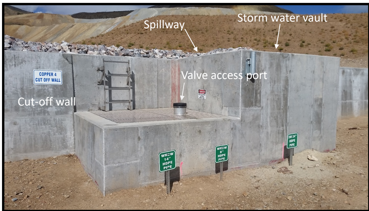
Figure 3-6. Photograph of a newly constructed cut-off wall. The valve port allows access to manipulate the WRCW flow valves.
