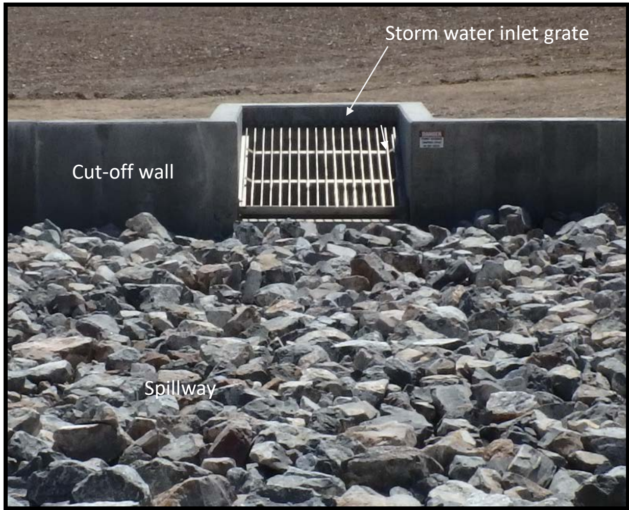
Figure 3-4. Photograph of a newly constructed spillway. The spillway connects the storm water detention basin to the cut-off wall.
