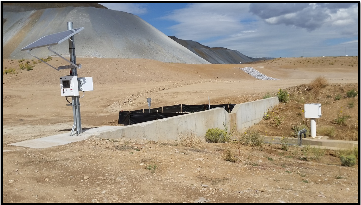
Figure 2-16. Storm water in the Copper 3 drainage connects to the lower concrete lined canal through a pre-existing storm water flume.
