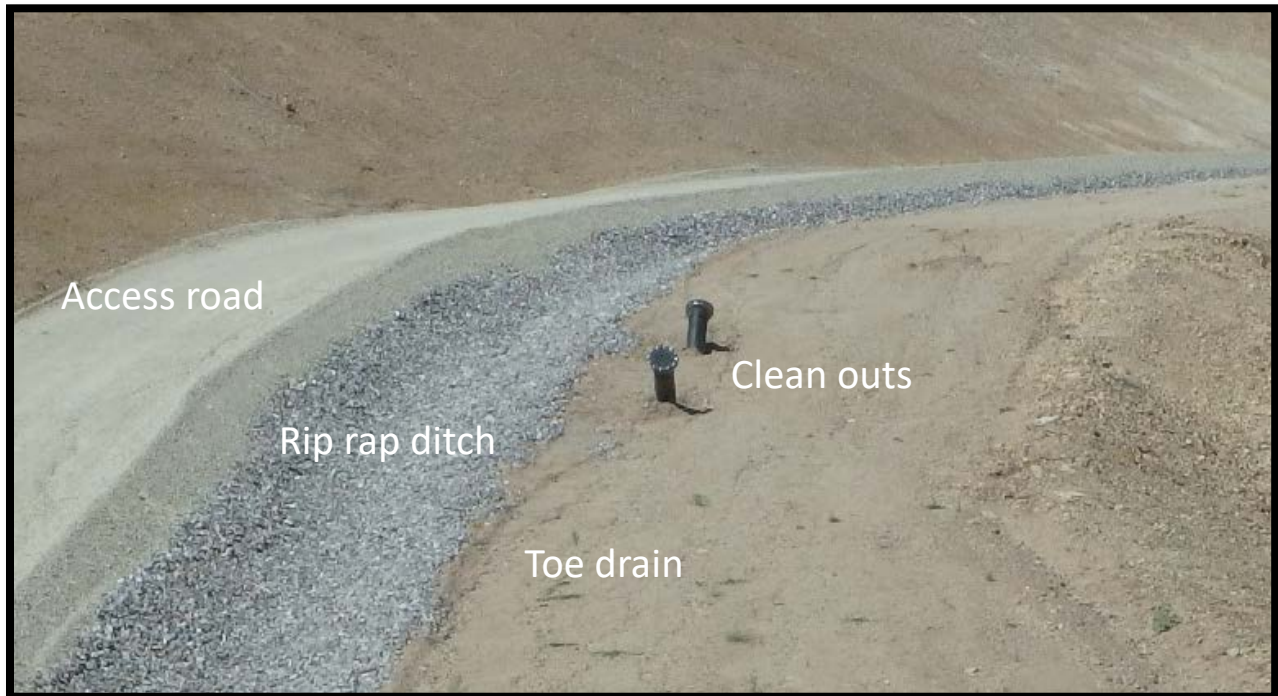
Figure 3-2. Photograph of a newly constructed segment of the toe drain; toe drain features include the clean outs, rip rap ditch and access road.
