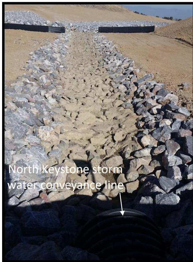
Figure 2-21. Photograph showing the 14-inch-diameter HPDE pipe conveying WRCW under the Mine Access Road in the North Keystone drainage basin. The coarse quartzite finger drain directs WRCW flow toward the North Keystone segment of toe drain.
