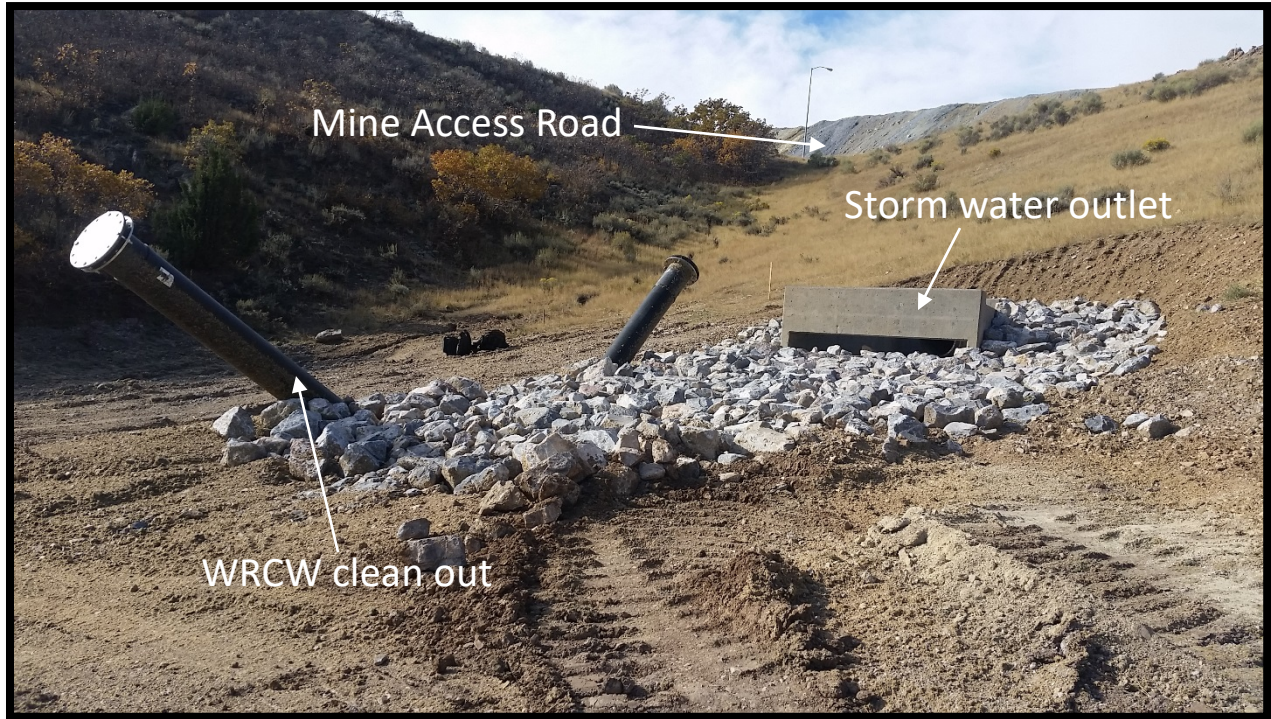
Figure 2-18. Lost Creek drainage directional boring outlet.
