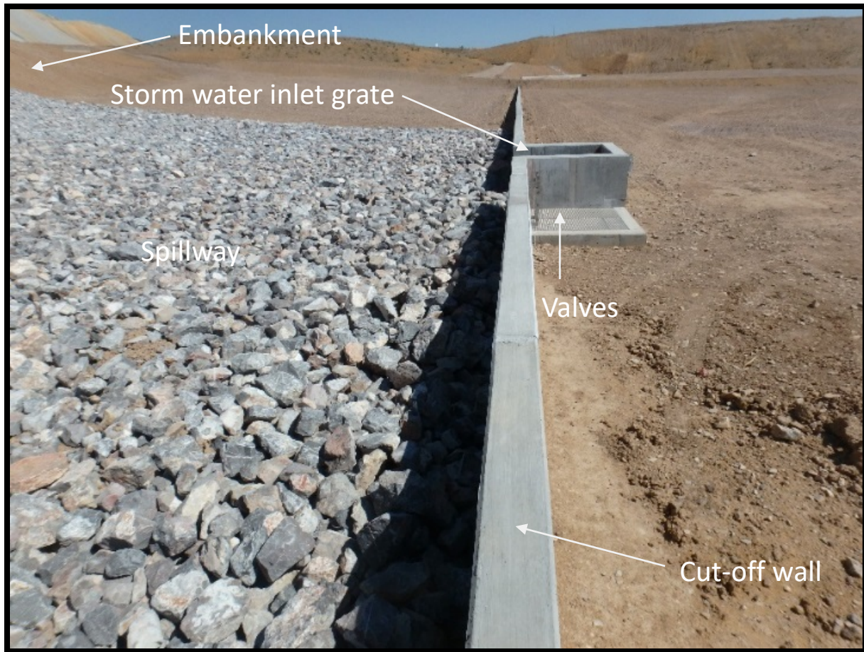
Figure 3-5. Photograph of a newly constructed cut-off wall. The spillway connects the storm water detention pond to the cut-off wall; the cut-off wall includes a storm water inlet grate and a valve vault.
