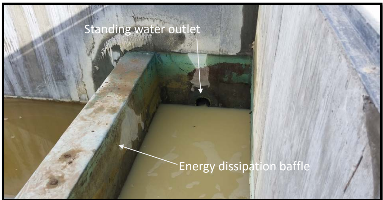
Figure 2-27. Storm water inlet structure by Copper 3.
