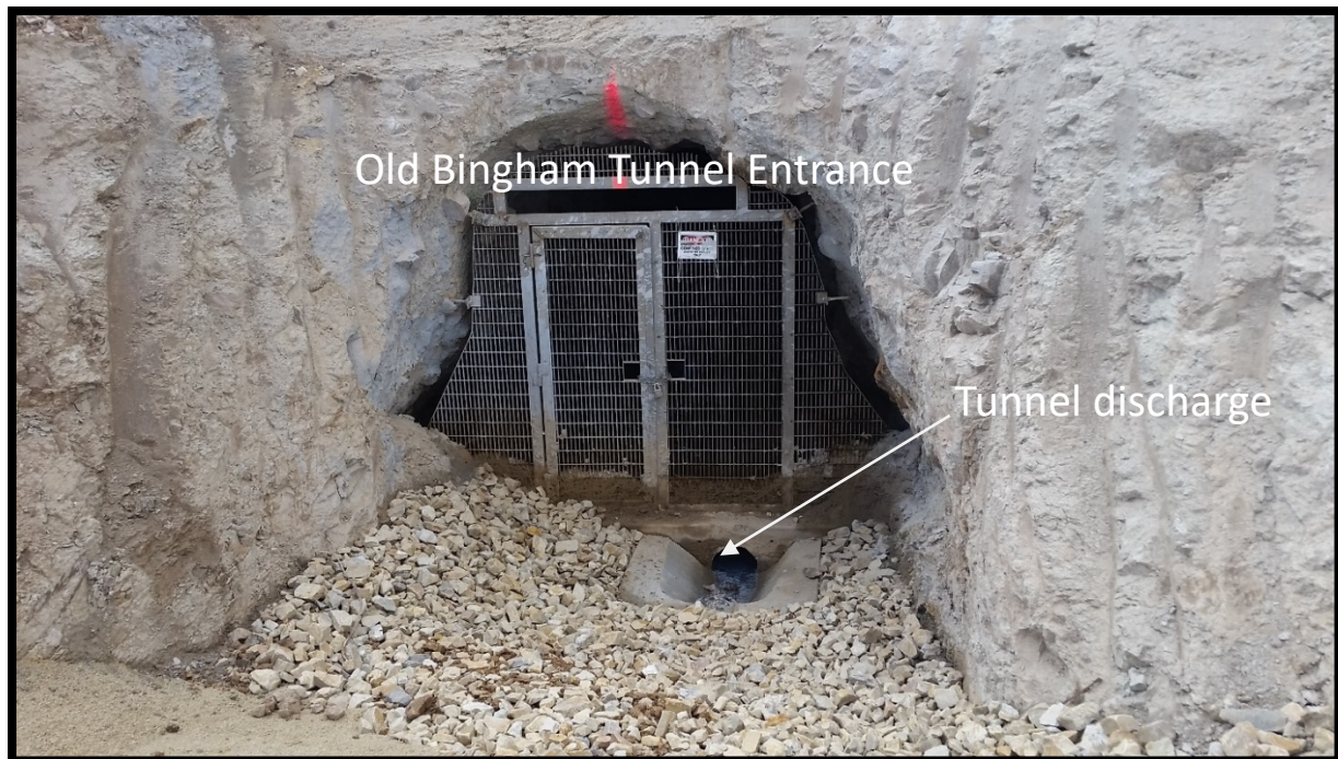
Figure 2-24. Photograph showing tunnel discharge from the Old Bingham Tunnel (OBT). The tunnel discharge from the OBT is conveyed to the combined South Congor and Midas weir box, but enters below the V-notch flow measuring point.
