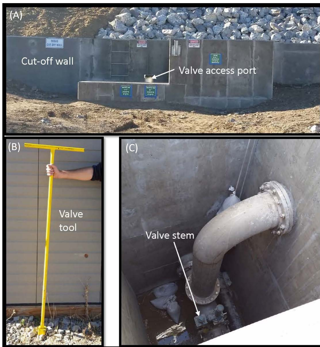
Figure 2-8. (A) WRCW by-pass valve located in each cut-off wall; (B) manipulated with valve tool; (C) valve tool attaches to valve stem for manipulation.
