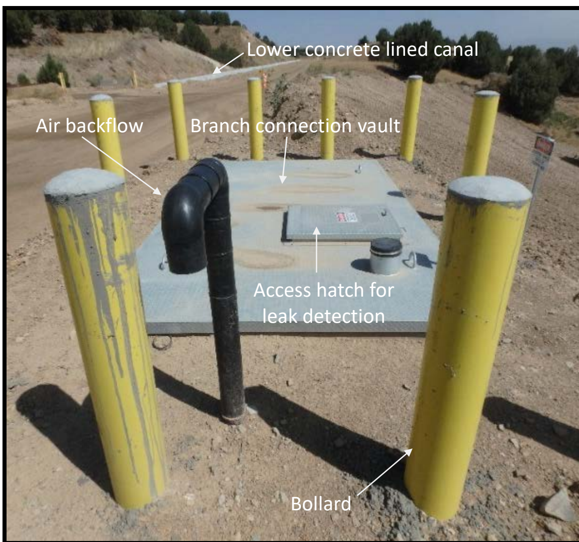
Figure 3-8. Photograph of a newly constructed WRCW branch connection vault.
