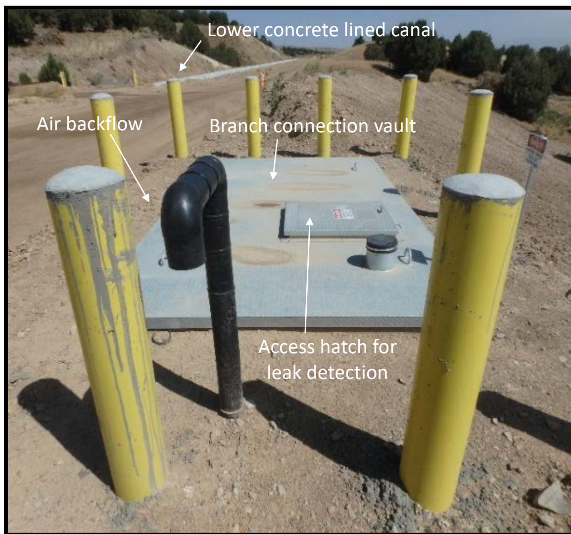
Figure 2-13. Photograph of a newly constructed WRCW branch connection vault.
