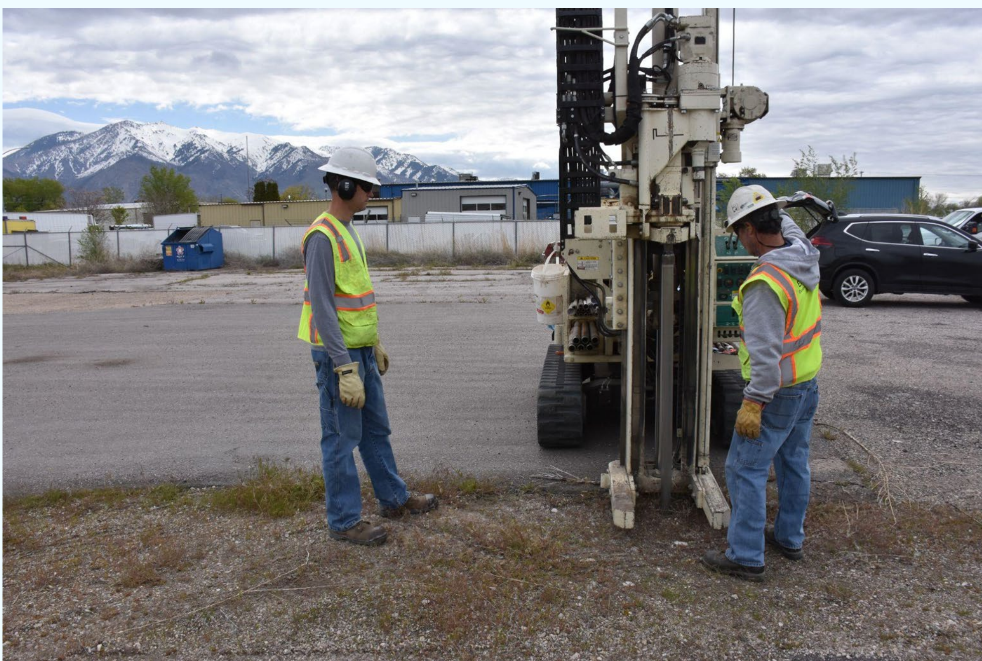
Drilling during soil and groundwater sampling at a closure.
