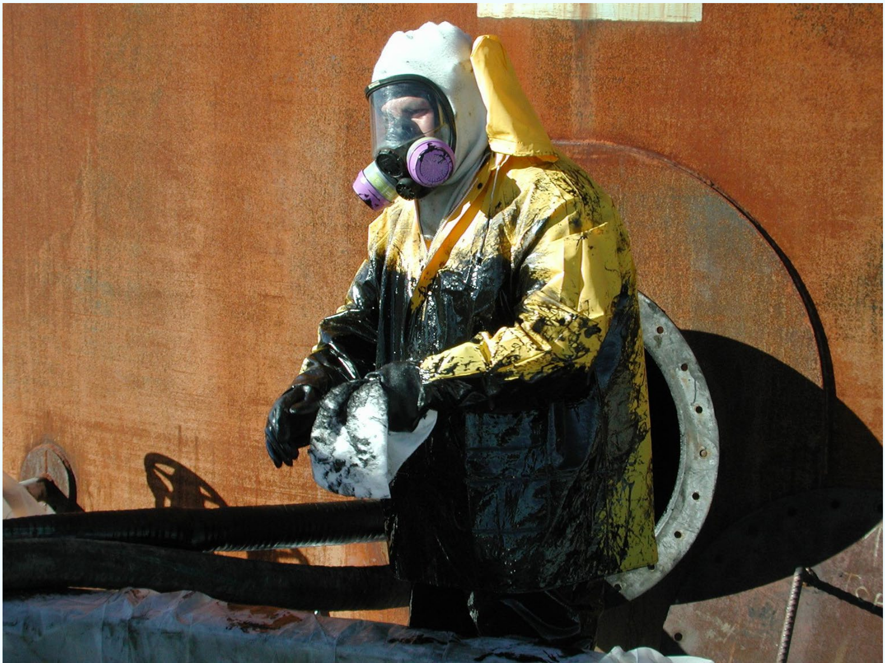
Cleaning out tank bottoms in Green River, Utah during closure.
