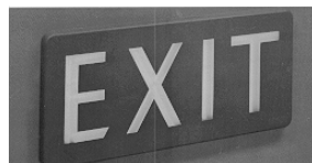
Figure 5-4. Tritium Exit Signs. Certain tritium exit signs can be possessed under 10 CFR 31.5 {typical devices contain 935 gigabecquerels (GBq) [25 curies (Ci)] of tritium per sign}.
