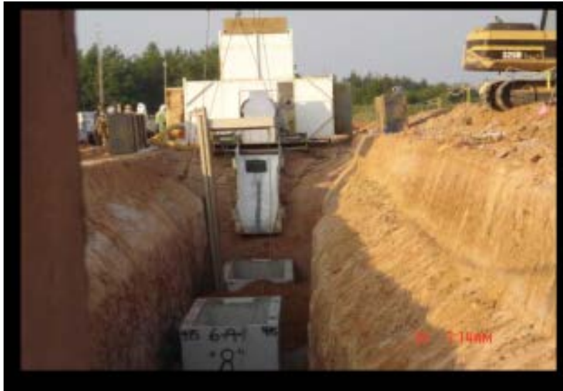
Figure C-15. Barnwell, SC Concrete Vault Placement
