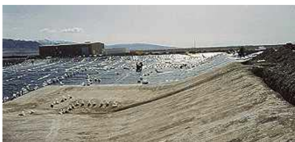
Figure C-21. Clive, UT Mixed Waste Liner Placement
