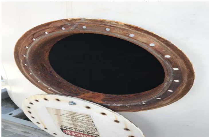
Manways / Nozzles - Flange condition
