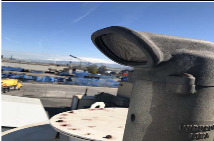
Roof Appurtenances - Condition of screens on vents
