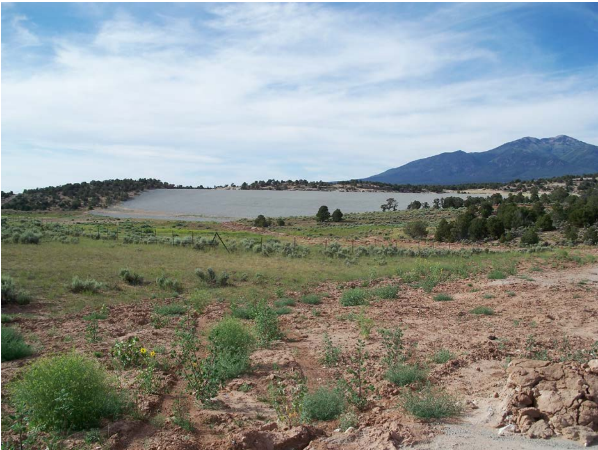
Photograph #1: The front of the Lower Tailing Impoundment. Showing the completed erosion barrier.
