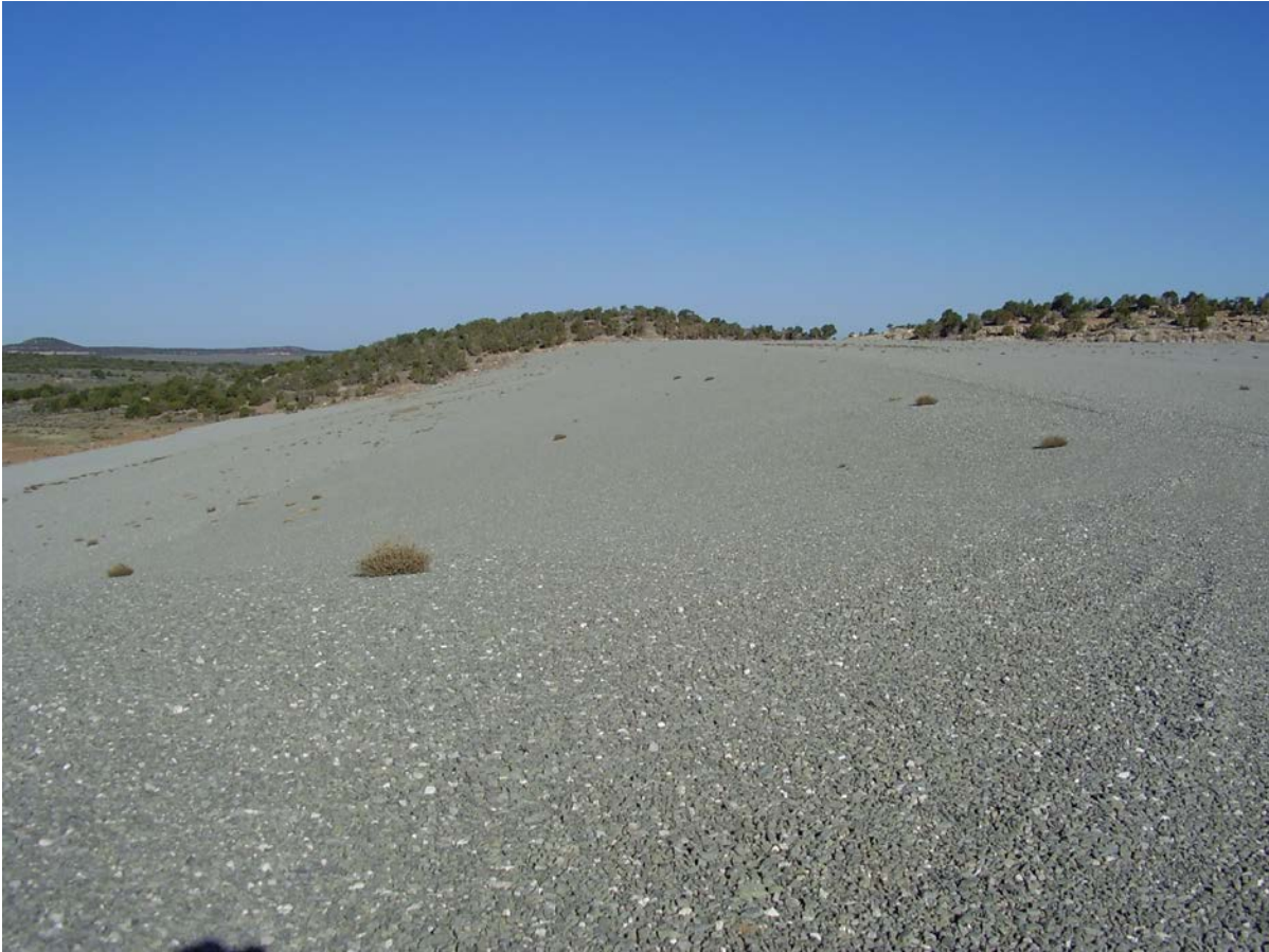
Photograph #3: The front and top of the Upper Tailing Impoundment. Showing the completed erosion barrier.
