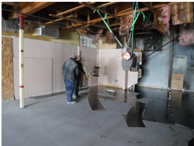
Photo 35 – Typical primer coat installation activities for the vapor barrier installation
