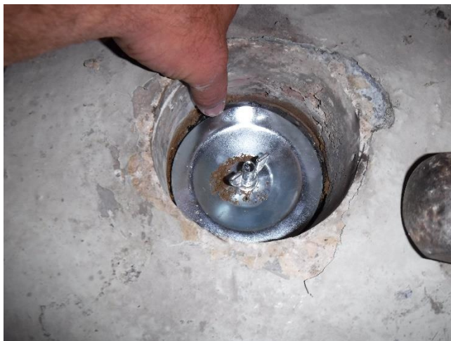
Photo 3 – Additional pipe plugged within the former Henries tenant space
