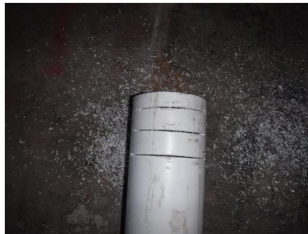
Photo 26 – Perforated portion of the passive vapor mitigation system
