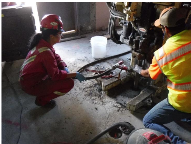
Photo 19 – Typical temporary injection well head inside former Henries tenant space
