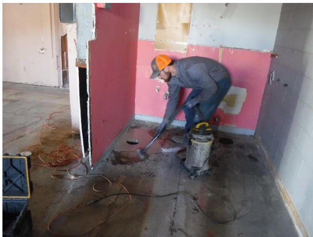
Photo 27 – Core hole for the vapor mitigation system
