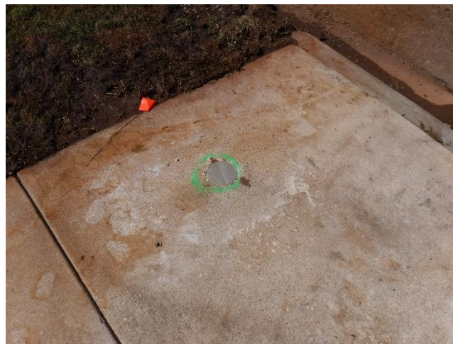
Photo 20 – Typical concrete patch post injection activities
