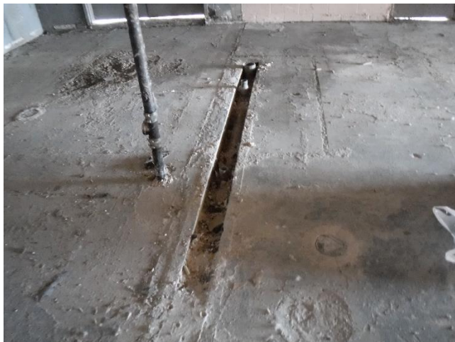
Photo 1 – Former drain pipe trench within the former Henries tenant space
