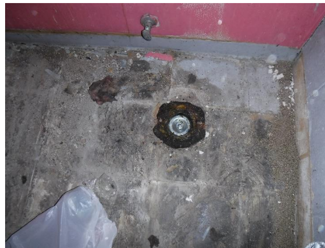
Photo 4 – Toilet drain plugged within the former Henries tenant space
