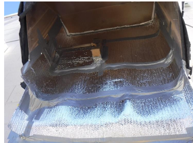
Photo 32 – Typical vent sealing to facilitate the vapor barrier installation
