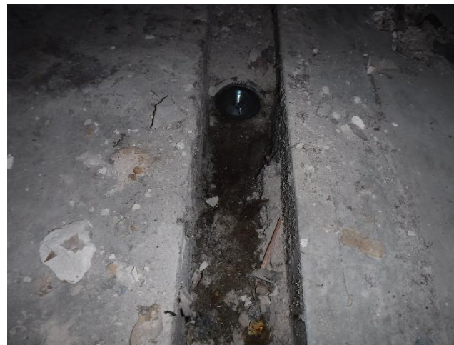
Photo 2 – Exposed trench pipe cut and plugged
