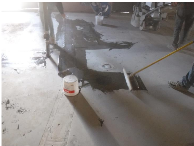
Photo 33 – Typical crack and joint filling activities for the vapor barrier installation
