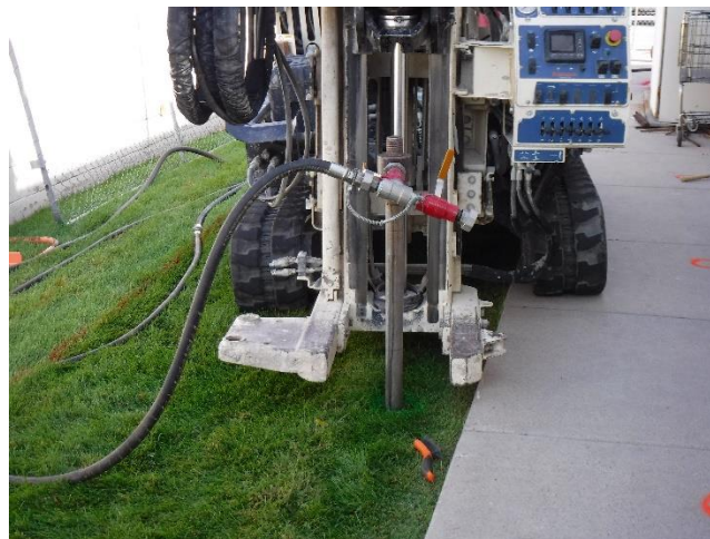
Photo 18 – Typical temporary injection well head
