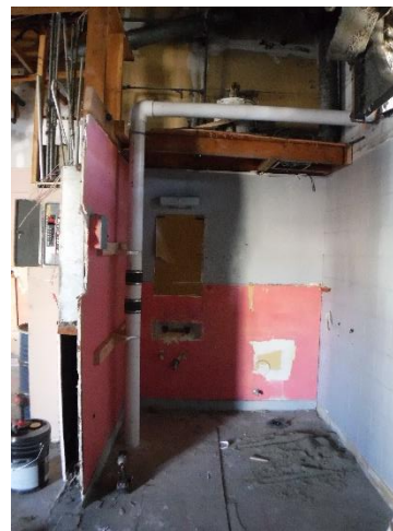
Photo 28 – Interior piping for the vapor mitigation system
