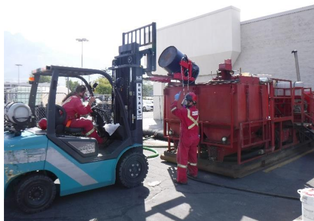
Photo 16 – Mixing ZVI for injections
