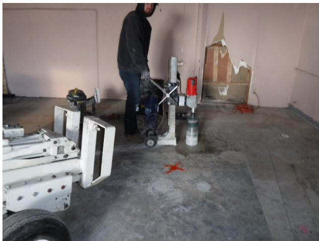
Photo 21 – Typical concrete coring for confirmation soil sampling activities
