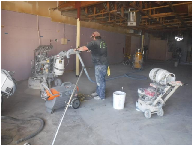
Photo 31 – Vapor barrier installation floor preparation
