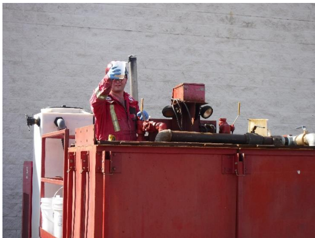
Photo 15 – Mixing gel for injections
