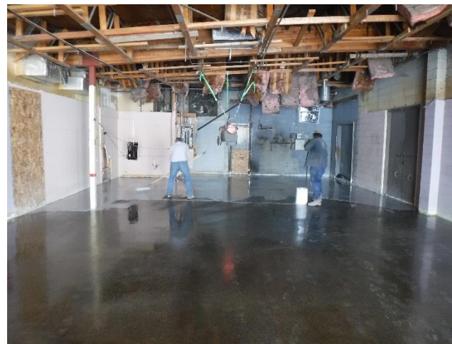
Photo 38 – Typical Retro-Coat installation activity
