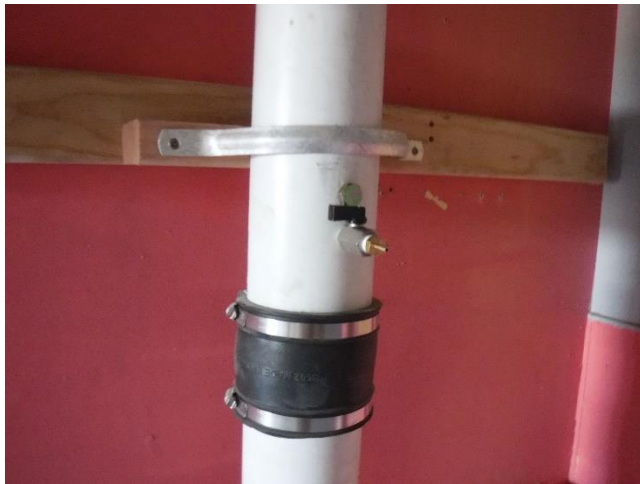
Photo 29 – Sampling ports for the vapor mitigation system
