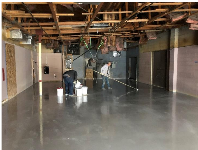
Photo 39 – Retro-Coat mostly installed
