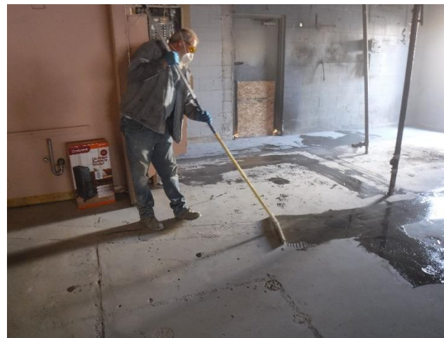
Photo 34 – Typical crack and joint filling activities for the vapor barrier installation
