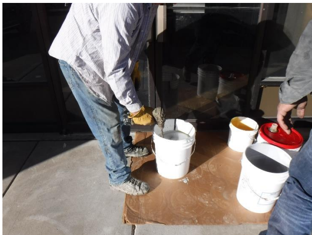
Photo 37 – Mixing Retro-Coat vapor barrier material
