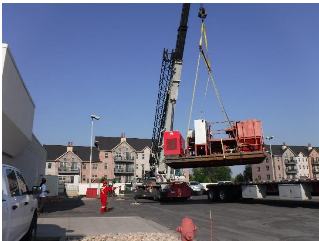
Photo 9 – Unloading the injection pump
