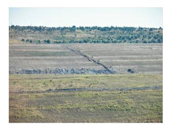
FIGURE 1 A large gully on a rehabilitated mine caused by concentrated flow collected on top of the landscape being greater than the capacity of the contour bank. Runoff erodes the bank and moves downslope to the next contour bank, which is also unable to contain the increased flow as a cascading failure and is common on mine sites [Color figure can be viewed at wileyonlinelibrary.com]
