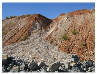
**FIGURE 4** (Top) Gullying on a post-mining landform with material placed at angle of repose. Runoff has collected on the flat cap and directed down the face of the unconsolidated material. (Bottom) Deposition is evident, which exerts base level control [Color figure can be viewed at wileyonlinelibrary.com]
