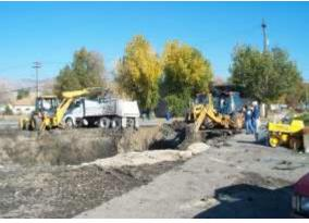
removal of the USTs and soil overexcavation activities. This resulted in significant construction and cleanup cost savings.
