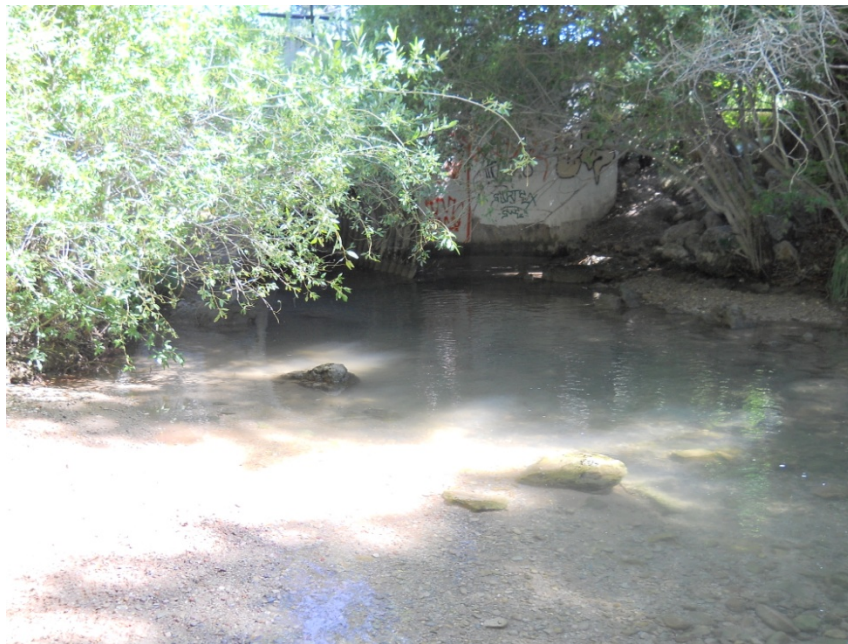
Photo 30: Parleys Creek below 1700 E, looking upstream at 1700 E culvert.
