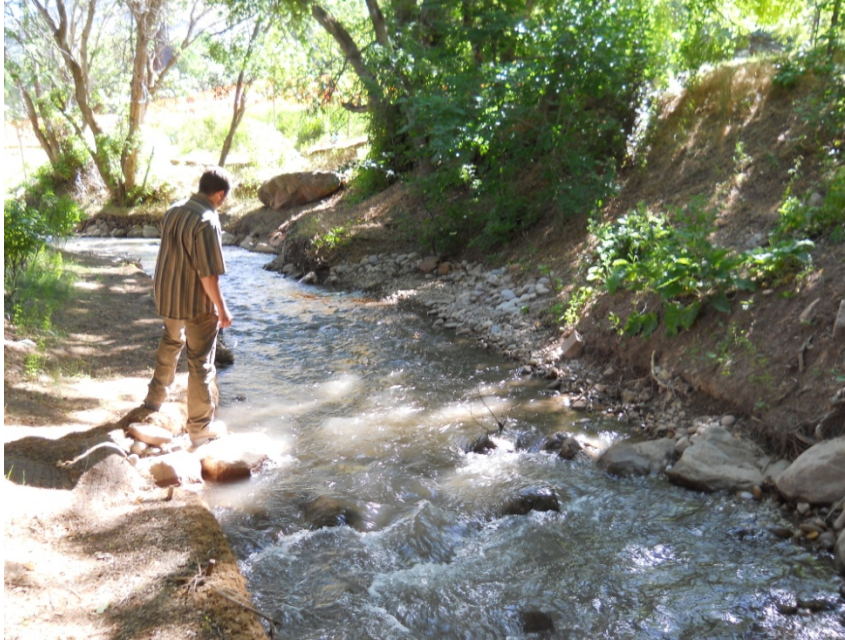
Photo 15: Red Butte Creek at Lower Underflow Dam, looking upstream. Creek channel here was reconstructed using all new bed material.
