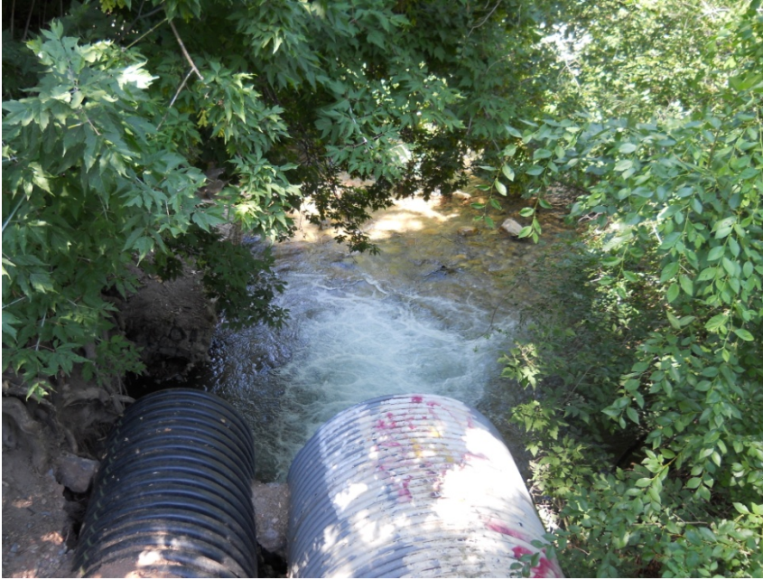
Photo 19: Mill Creek below 2300 E.
