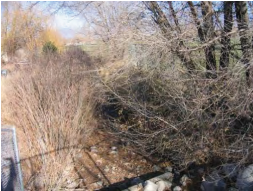
Photo No.5 – Bingham Creek channel 2700 West, view to east.
