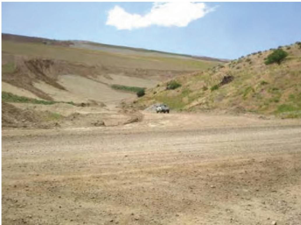
Photo No. 30 – View up Bingham Canyon illustrating the extent of encroachment of mine waste deposits. All historic facilities in this are (OU11) have been buried by mine waste deposits. View to West.
