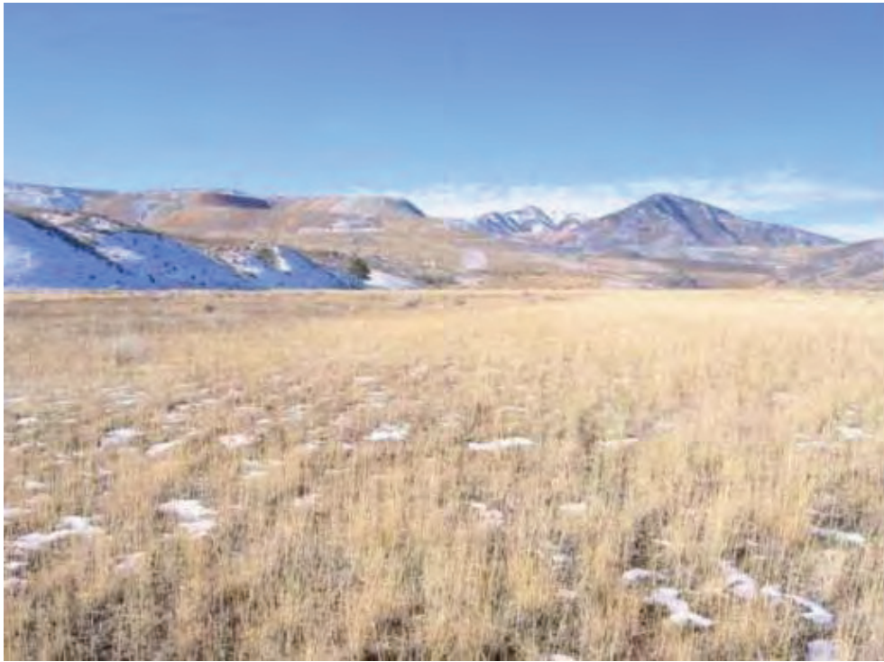
Photo No. 23 – Top surface of the tailings repository (looking west). The photo was taken to document the planting rows still visible from the revegetation efforts in 1997. 12 years have expired since the revegetation effort and these rows help to document the stability of the cap on the repository.
