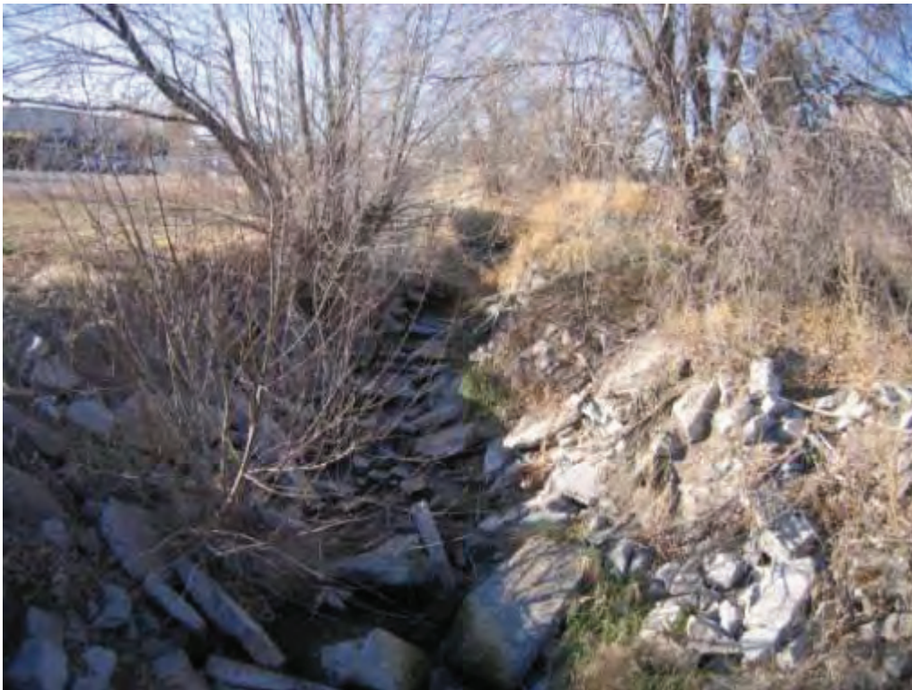
Photo No.2 – Bingham Creek channel 1300 West, view to the west.
