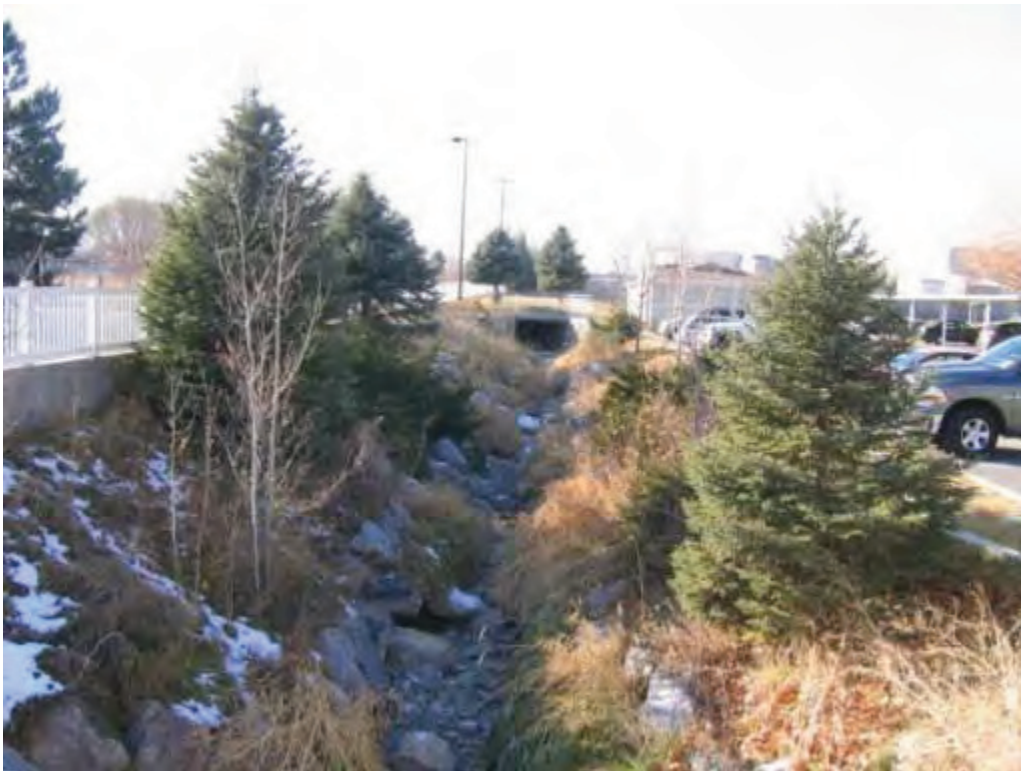
Photo No.6 – Bingham Creek channel near 2700 West, view to the west.
