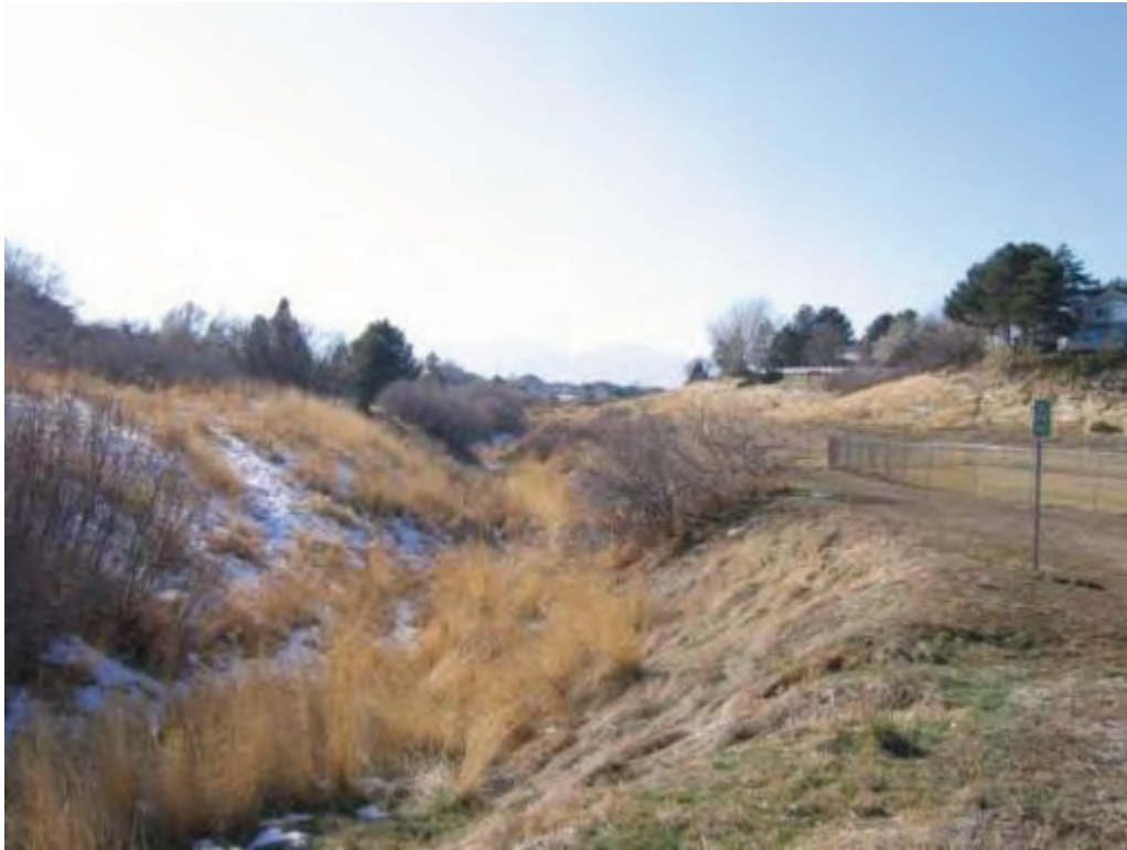
Photo No.10 – Bingham Creek channel near 4400 West, view to the west.
