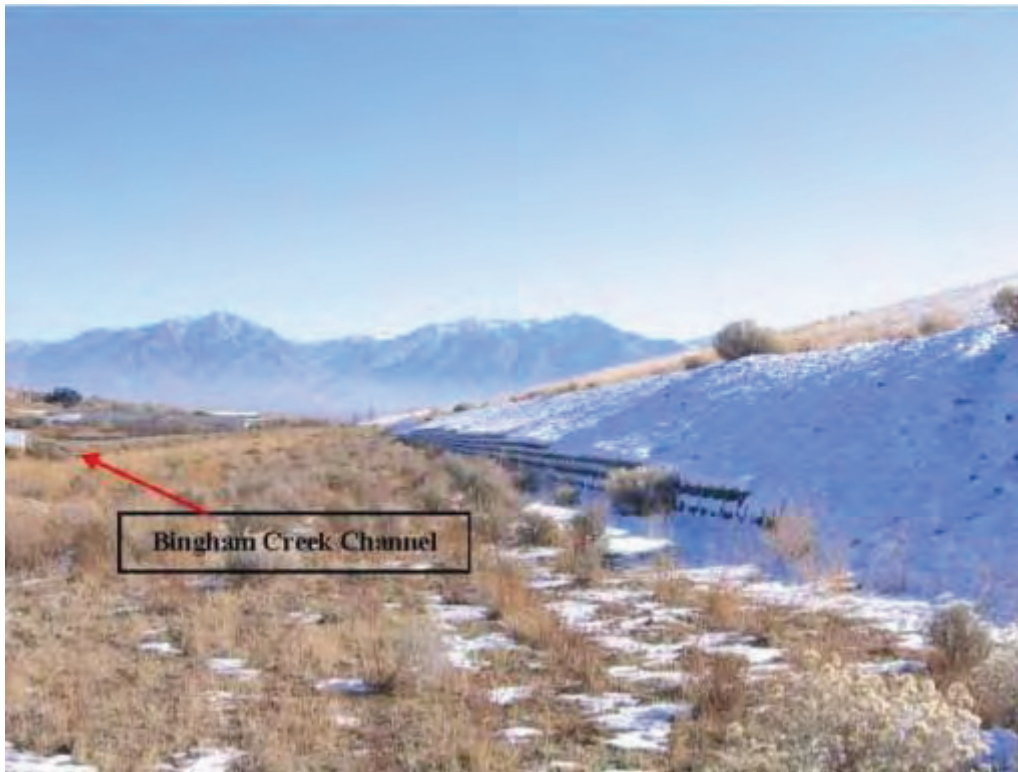
Photo No. 26 - Northern embankment of the tailings repository at OU5 viewed from the northwest corner.
