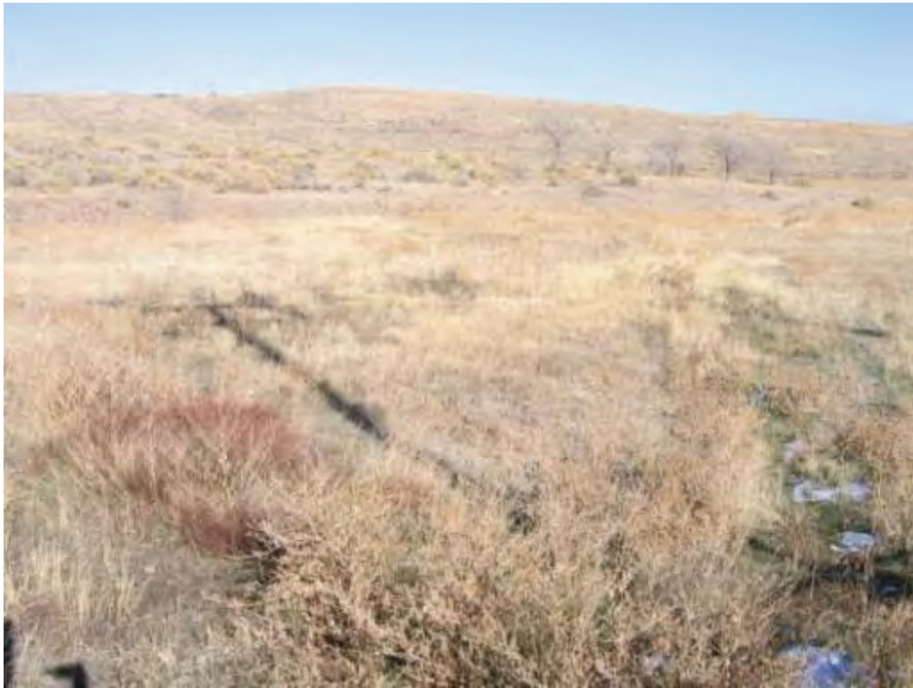
Photo No. 29 - Area of the buried drainage pipe leading off to Bingham Creek Channel (after Repair).
