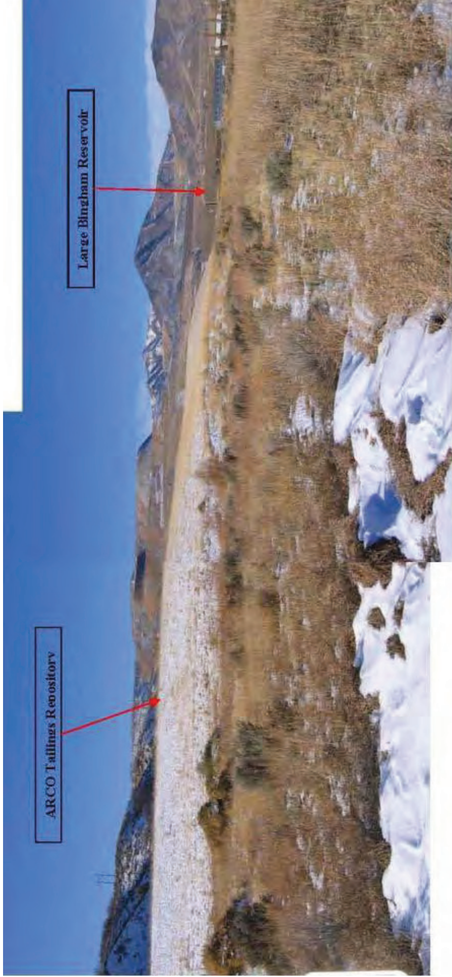
Photo No.18 – Top and east slope of repository. The top of the repository is sloped to the south/southeast. The slope was stable, with very little erosional activity along it.
