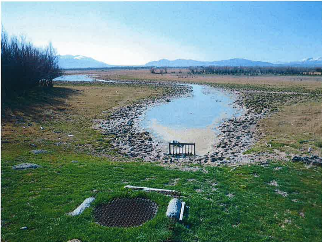
Photo 3. View from the top of dike looking south; below is the old control structure.
