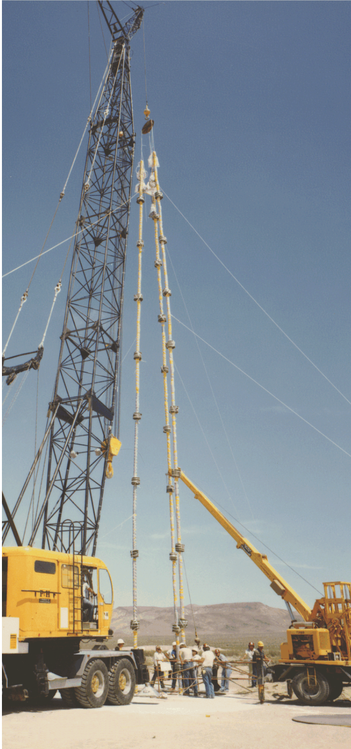
Figure 1-6. Placement of Monitoring Equipment in the GCDT Borehole.
