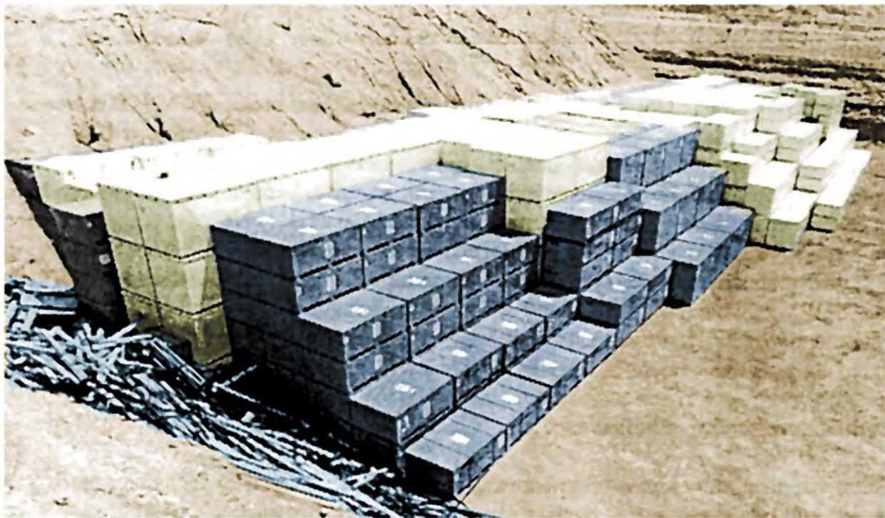
Figure 2.1. Waste Container Emplacement in a Typical Trench, Area 5 RWMS.
