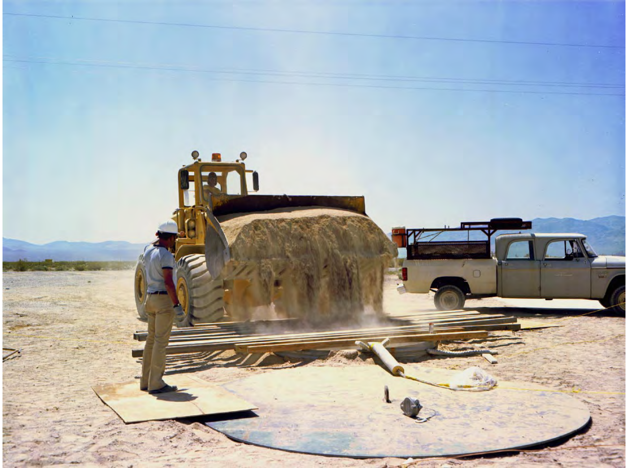
Figure 2.4. The Backfilling of the GCD Borehole.
