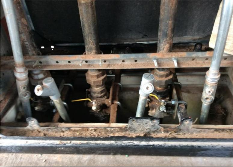
This picture is taken from underneath a dispenser. The presence of ball valves (see yellow handles), underneath breakaway valves, invalidates the breakaway valves. The ball valves need to be replaced with a proper plug from the respective manufacturer. This is a safety issue.
