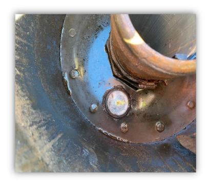
This is a picture of a spill bucket gauge that indicates there is liquid in the interstices. To correct this, it needs to be cleaned out and pass a tightness test. Either a hydrostatic or vacuum test.
