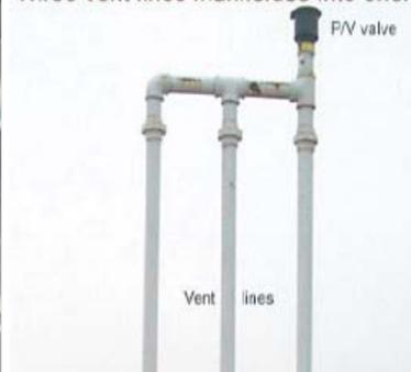
Three unmanifolded vent lines with three P/V Valves.
