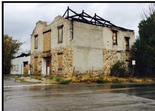
Brigham City - Merrell Planing Mill Site
