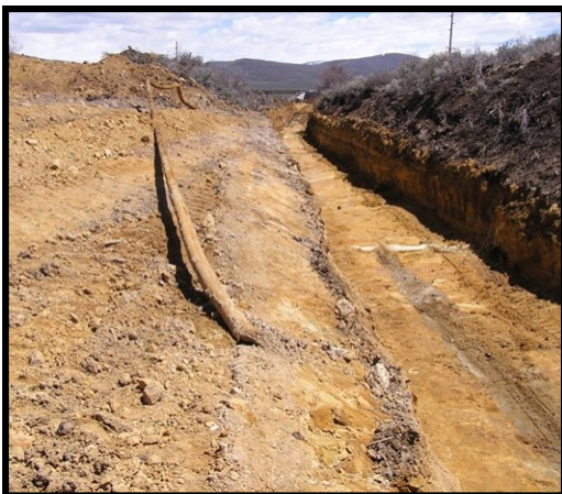
Removal of impacted soils
