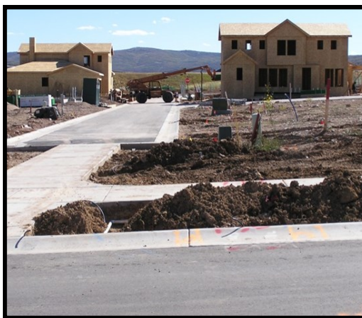
Construction of a residential subdivision
