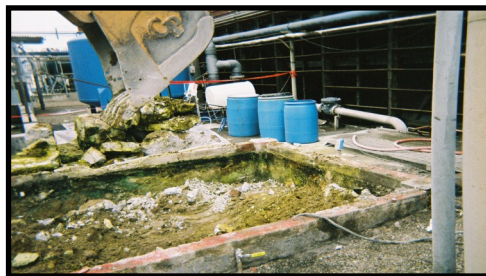
Geneva Nitrogen Site Remediation - Vineyard
