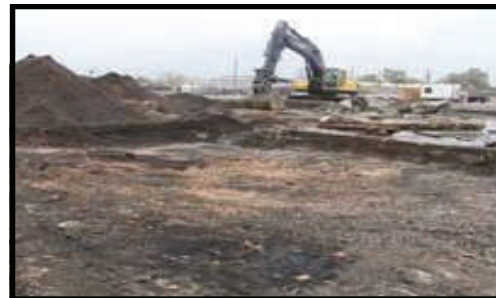
Removal of contaminated soil from the Utah Barrel and Scrap site. From Left to Right: October 2008, soil removal and November 2008, excavation.
