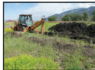
Trenching into the landfill cells under the retention basin.
