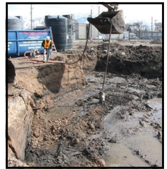
Soil excavation at the 300 West Town Center.
