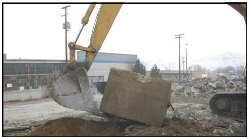
Underground waste vat found and removed.
