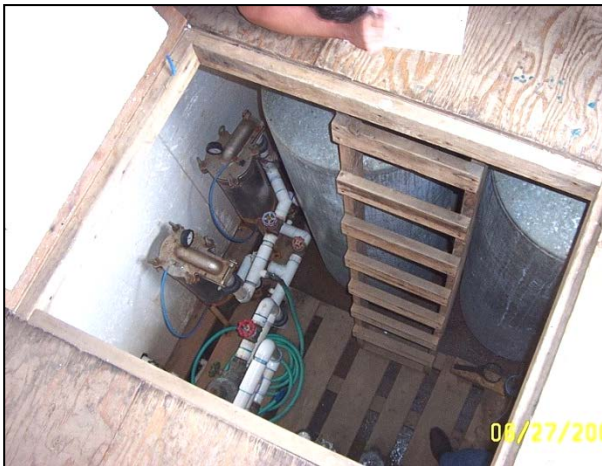
Well and Filter Vessels Located in a Pit with Unsafe Access Ladder
