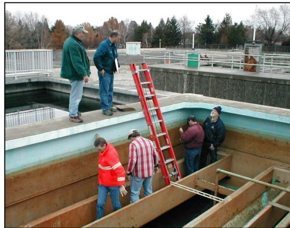
Gravity Rapid Sand Filter Basins
